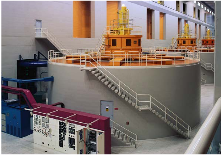
These dam generators use the force of river water to spin magnets and make electricity.
